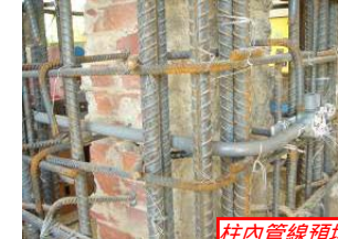
柱內管線預埋
