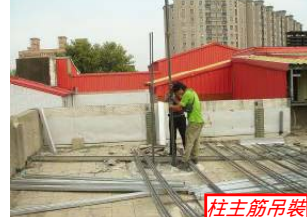
柱主筋吊裝
