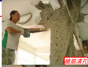
柱梁接頭植筋鑽孔
